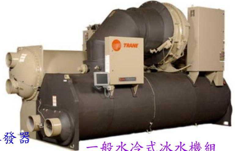
Figure 2 Dual-condenser heat-recovery centrifugal chiller
